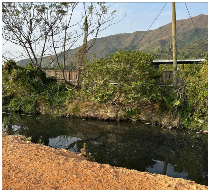
VIEW 2 Final Discharge Point
